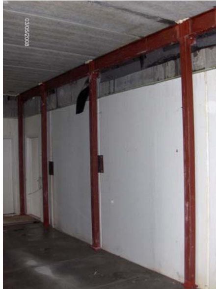
Figure 10. Photo (5 July07) of the steel construction in the building.
